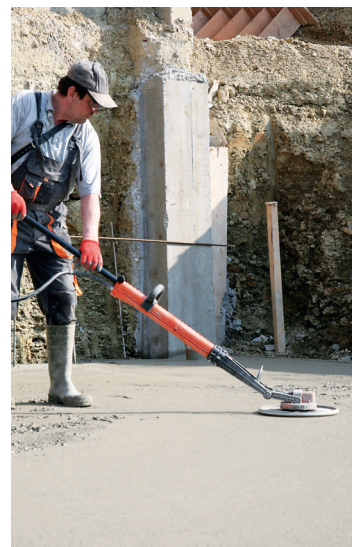
Levelling fresh concrete
